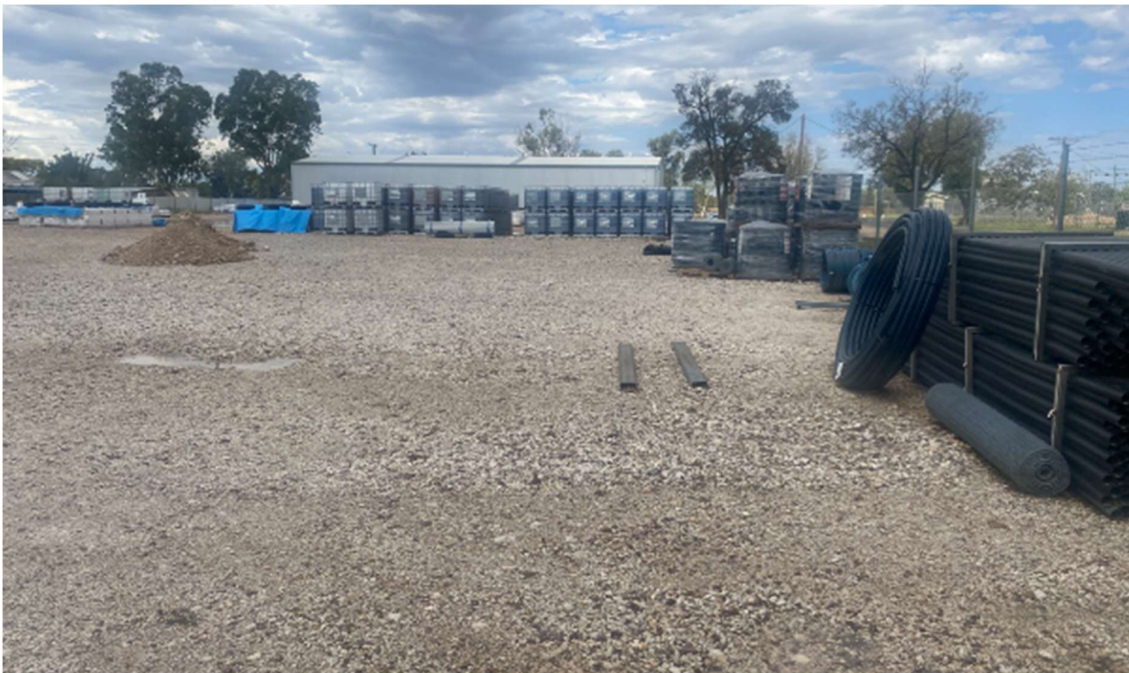
Figure 8: Gravel (“white rock”) pad established on Lots 8 and 9.
