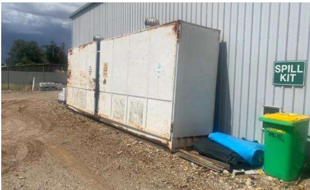
Figure 16: DG Storage container for Class 6.1 chemicals in the Chemical Storage Yard.
