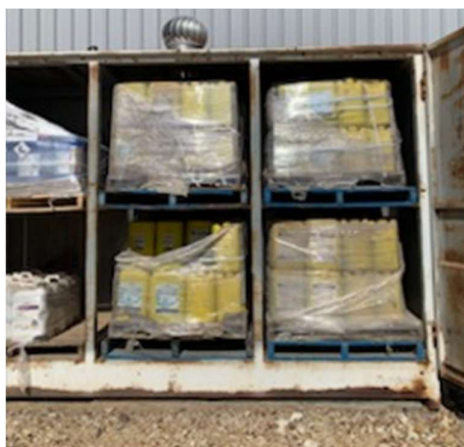
Figure 17: Existing DG container for Class 8 chemicals in the Chemical Storage Yard.
