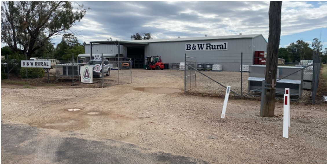
Figure 3: Existing Shed and Yarouah St entrance.
